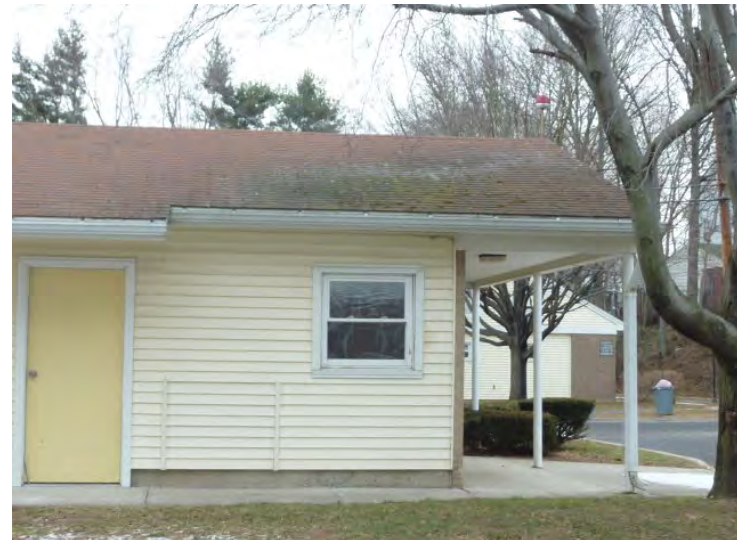
Asphalt roofing is in poor condition and is shown to be replaced at all 8 buildings.
