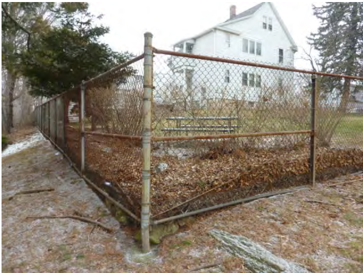
Chain link fence installed on the property line is rusted.
