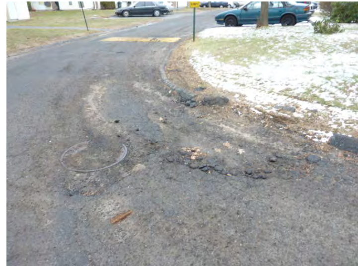
Typical asphalt paving sub-base failure.
