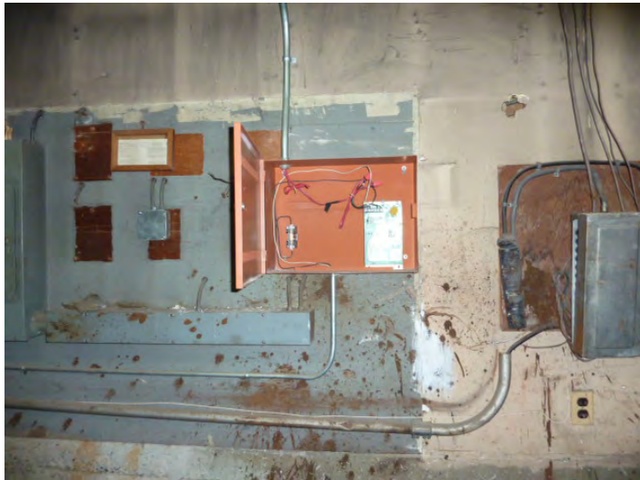
Community Center fire alarm control panel is shown to be upgraded.
